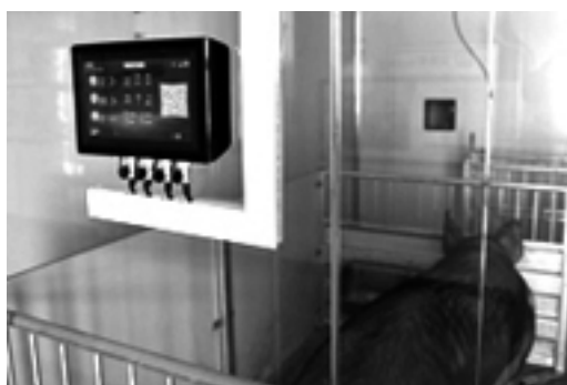
An automatic temperature and humidity controller at a pig farm in Jiaying, China.
